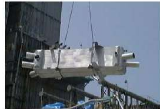
Braze aluminum plate-fin heat exchanger
